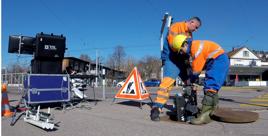
Fig. 4: Depiction of the field test setup and the deployment of ANYmal into the sewer. The operator base station and warnings signs are visible in the background.
