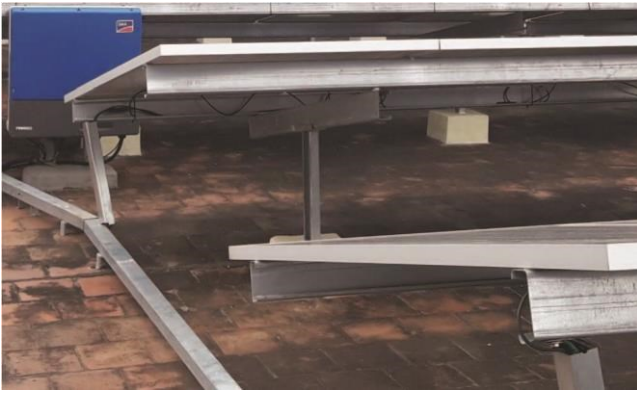
used for PV installation location the PV Watts shows the superior performance than
