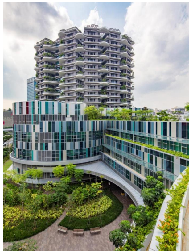
Fig. 25. Active use of landscaping in hospitals Ng Teng Fong (NTFGH) & Jurong (JCH). Source: https://www.wsp.com/en-MY/projects/ng-teng-fong-general-hospital-singapore
