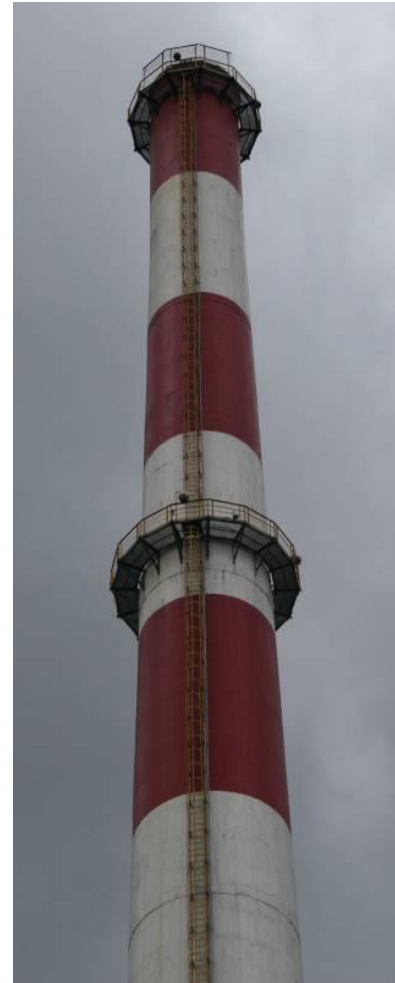
Figure 4b. Chimney after repair
