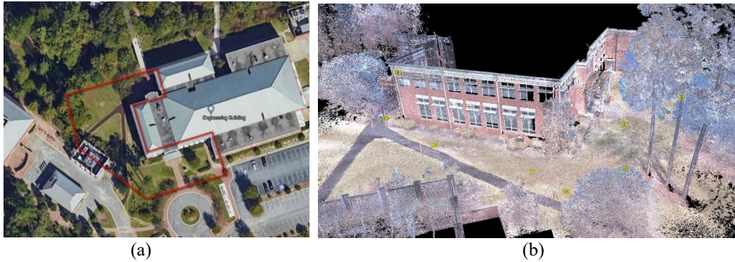
Figure 1. (a) Plan view of modeled area, marked in red, of Engineering Bldg. Picture from Google Maps, 2021. (b). Resulting Virtual, 3D, Point-Cloud Model (perspective view)
